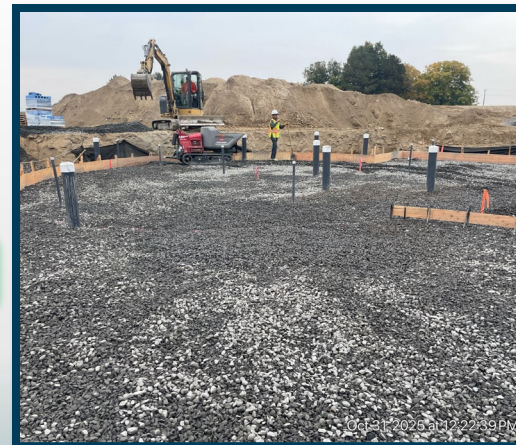
Pool Slab Rock Prep
