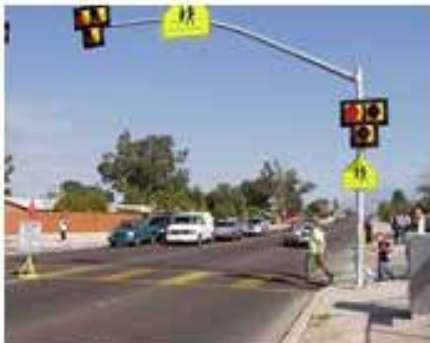
E) Signalized Crosswalk
