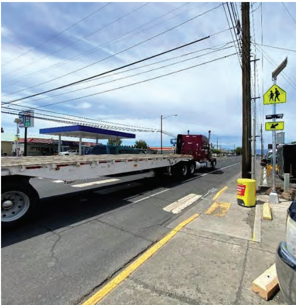
State Route 28 through Quincy is heavily trafficked, but some existing sidewalks are narrow and only separated by a small shoulder, such as this example near 3 rd Ave SW.
