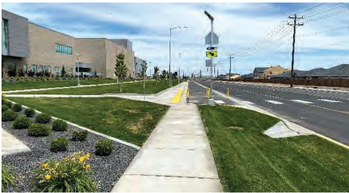
Sidewalks on Jackrabbit Street near Quincy High School offer landscaping buffers and crossings have flashing beacons to provide extra safety for students accessing the high school.
